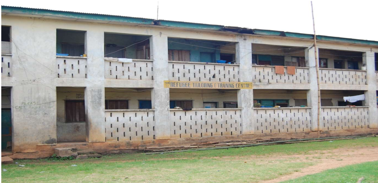
Figure 2: Skill Acquisition Building at Oru-Ijebu Refugee camp
